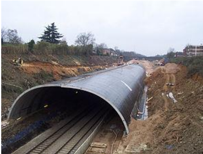
Figura 8 Excavación "Cut and Cover"
